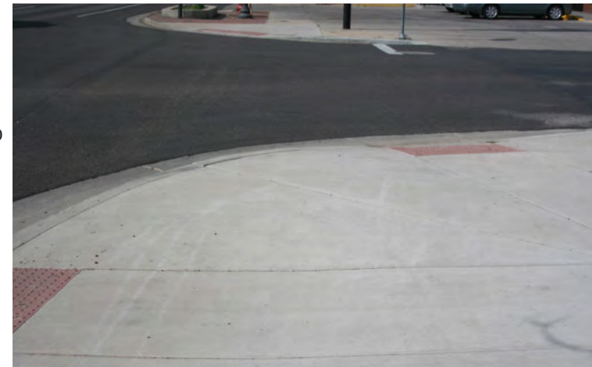
Fig 14: Existing Conditions - Blended Transition ADA Ramp
