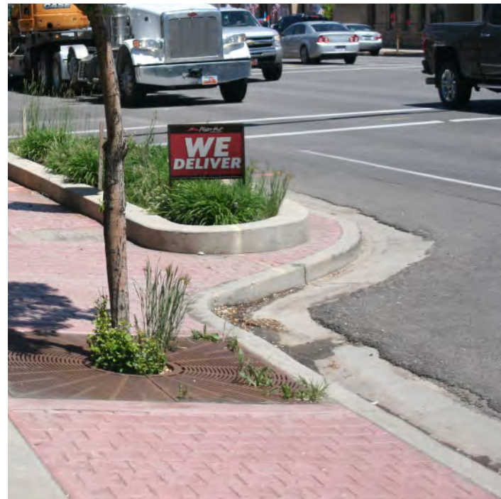
Fig 11: Existing Conditions - Deteriorated Curb and Gutter
