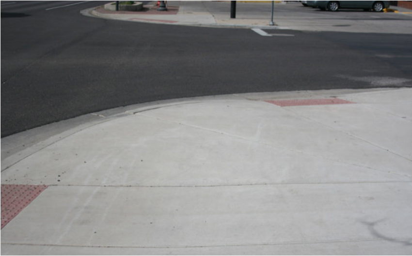
Fig 14: Existing Conditions - Blended Transition ADA Ramp
