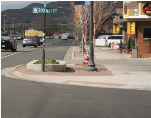
Fig 15: Existing Conditions - Separated ADA Ramp
