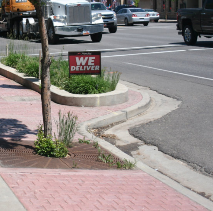
Fig 11: Existing Conditions - Deteriorated Curb and Gutter
